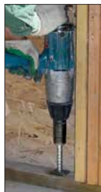
Suitable for use in place of code anchor bolts.
